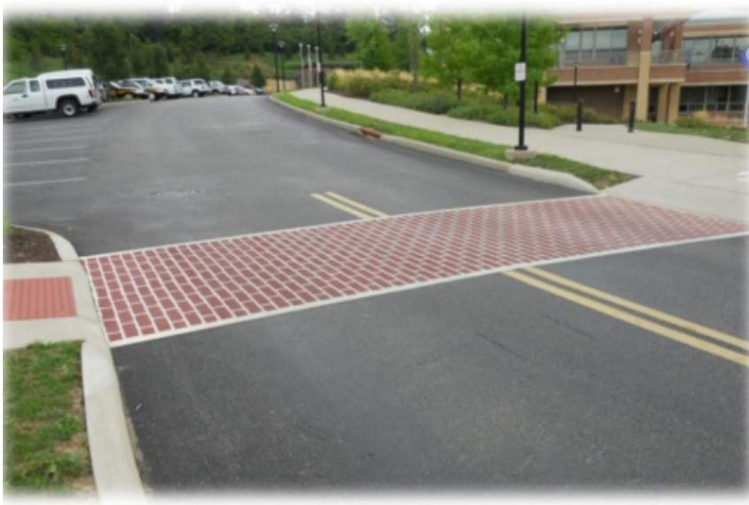
Elements such as stripping or pavement patterns can be used for aesthetics as well as traffic calming
